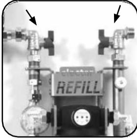
Close ball valves. Place a bucket below the cartridge.
